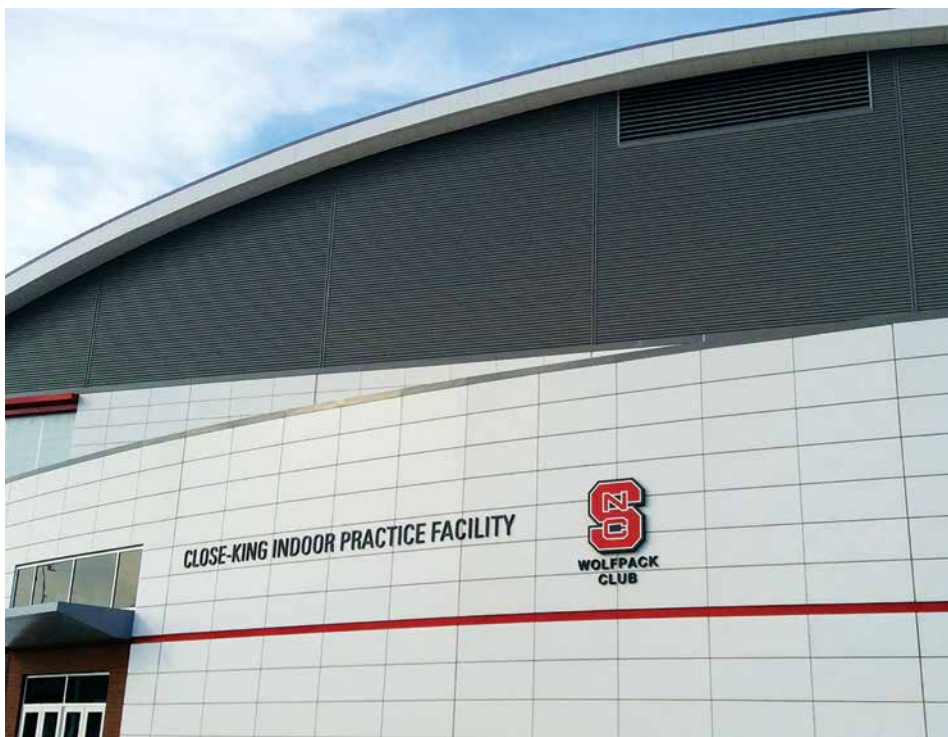
Close-King Indoor Practice Facility - LE-33A
