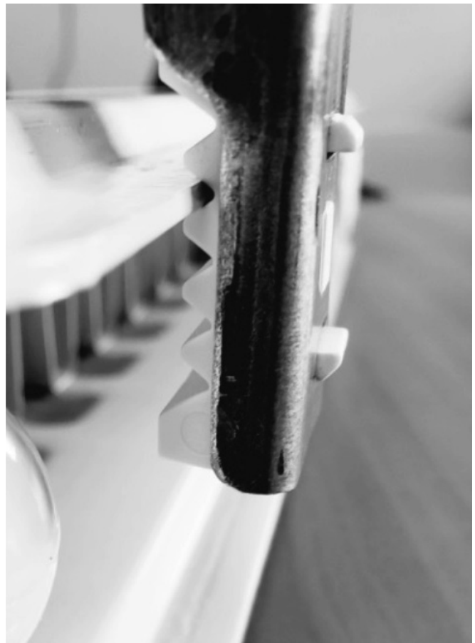
Figure 11 – J Bracket Bottom Notch installation
