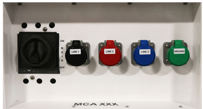
Figure 4 – Camlock & Circuit Breaker
