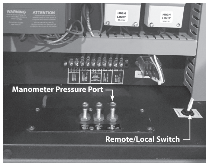
Figure 22 Manometer connections to manifold
