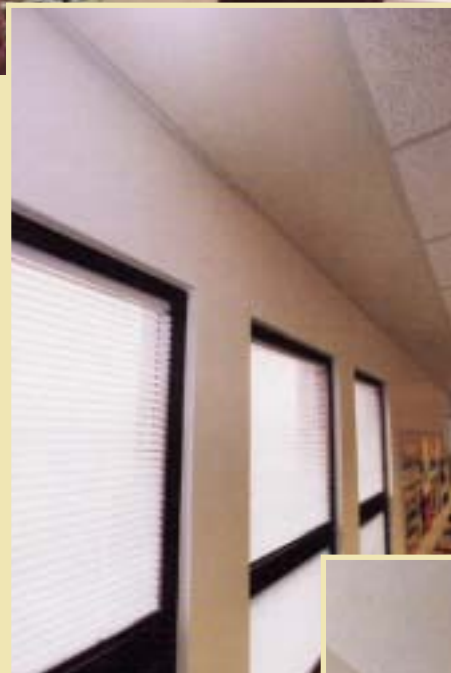
Panel placement provides comfort next to windows.
